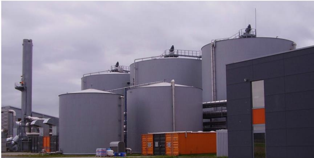
Figure 13: Anaerobic digestion unit in a Mechanical-Biological Treatment Plant in Germany.
